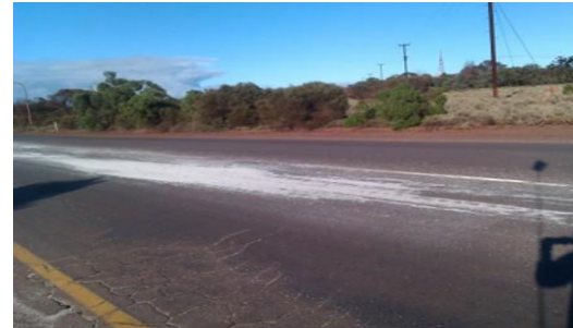
Spillage on roads
